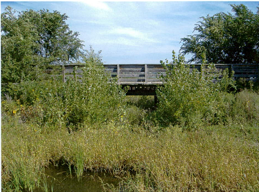
Photo 2: View of the old railroad bridge and bike path upstream of the Highway 50 culvert.
