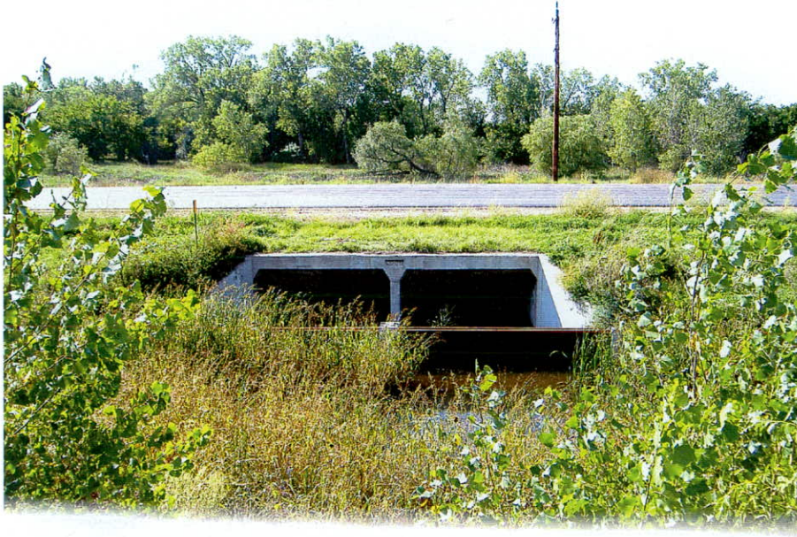
Photo 1: View of the Highway 50 Culvert from Lake Andes.
