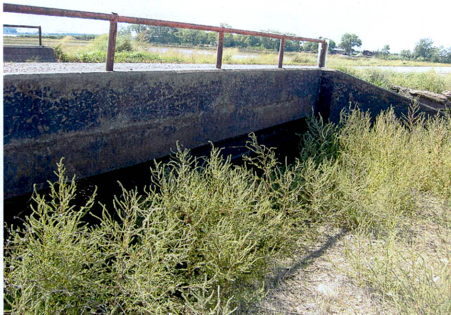
Photo 4: View of the upstream side of the South Dike bridge crossing.
