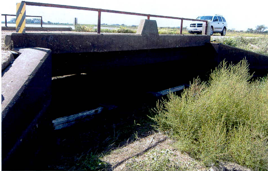
Photo 3: View of the upstream side of the North Dike bridge crossing.
