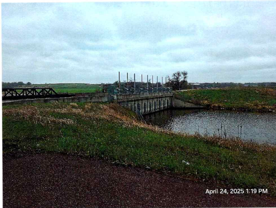
Big Sioux River Diversion Dam located in the NE \frac{1}{4} NW \frac{1}{4} Sec 32 T102N-R49W.
