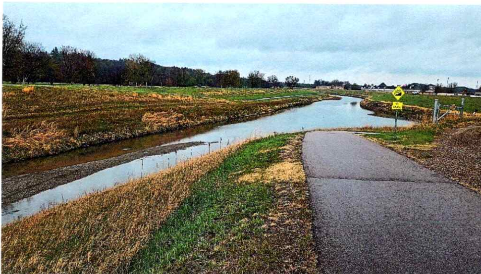
Big Sioux River channel levee raise located in the NE \frac{1}{4} Sec 25 T101N-R50W at the confluence of the Skunk Creek with the Big Sioux River.
