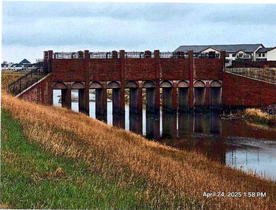
Big Sioux River a gated control dam upstream of the Skunk Creek confluence located in the NE \frac{1}{4} NE \frac{1}{4} Sec 25 T101N-R50W.
