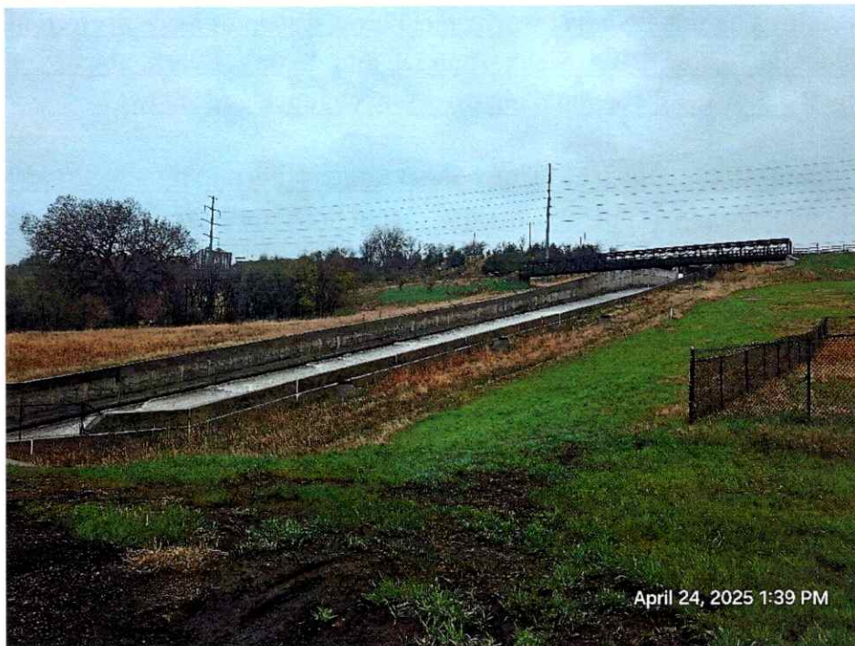
Diversion channel spillway located in the SE \frac{1}{4} NW \frac{1}{4} Sec 9 T101N-R49W.
