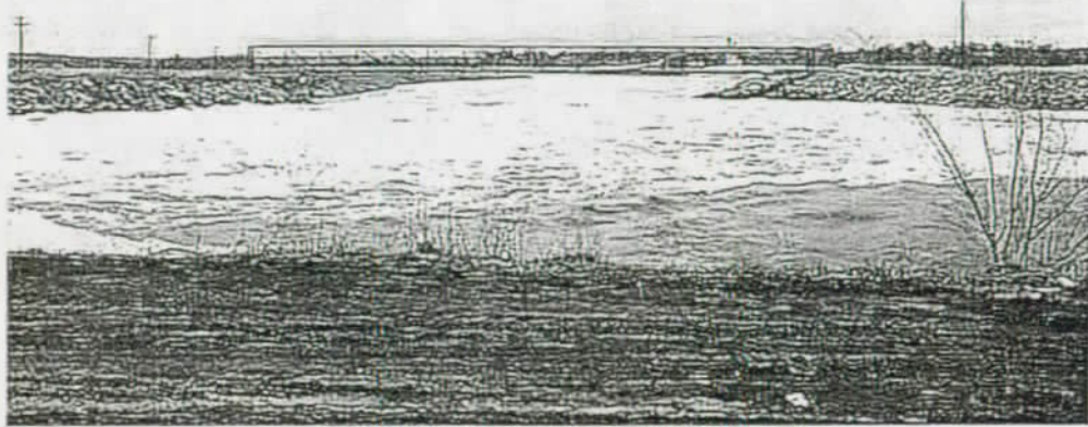
Exhibit 4 – Stilling Basin (1997 Flood)
