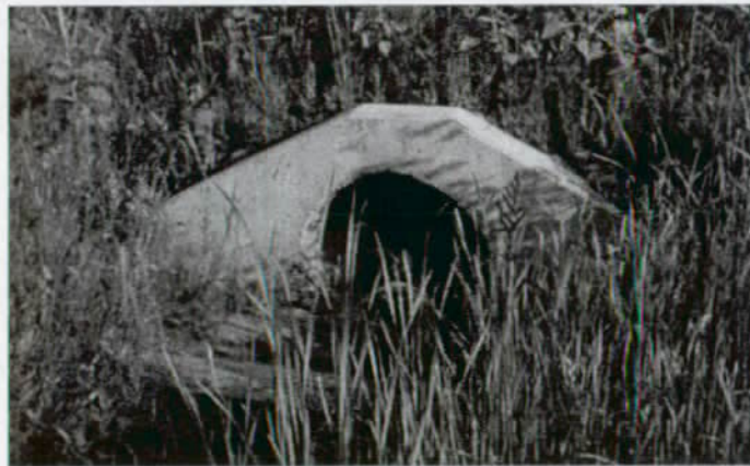
Inlet Structure for FC-17
