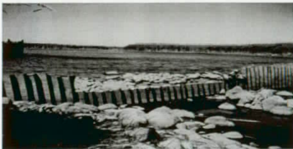
Figure 1. The 1' X10' notch in the sheet pile dam crossing the Big Sioux River. (1996)
