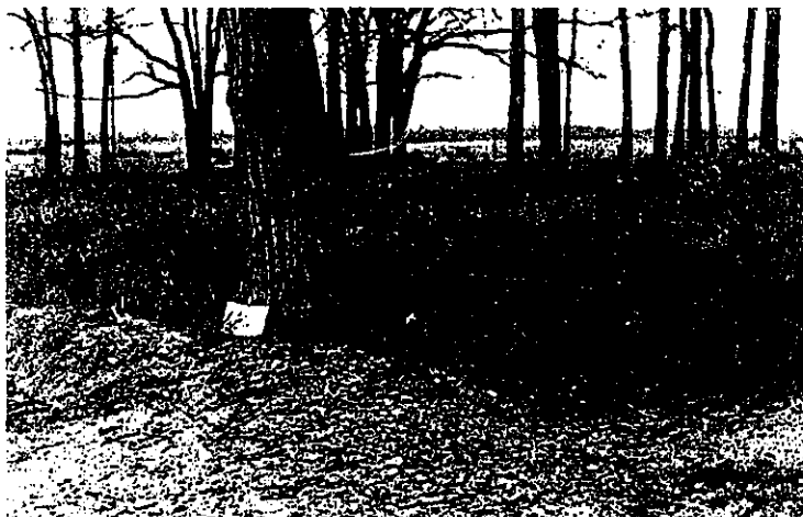
PHOTO NO. 7 Description: Cottonwood, Dia. 1.5 ft, Age 60 years Base Elevation: Lakeside----1824.0 Landside----1824.6
