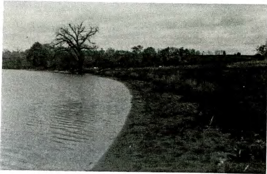
PHOTO NO. 10 Erosion Line Elevations (left to right from tree) 1802.2 1802.3 1802.3 1802.6 1802.3 1802.4 1802.3 1802.5 1802.1 1802.5 1802.4 1802.6
