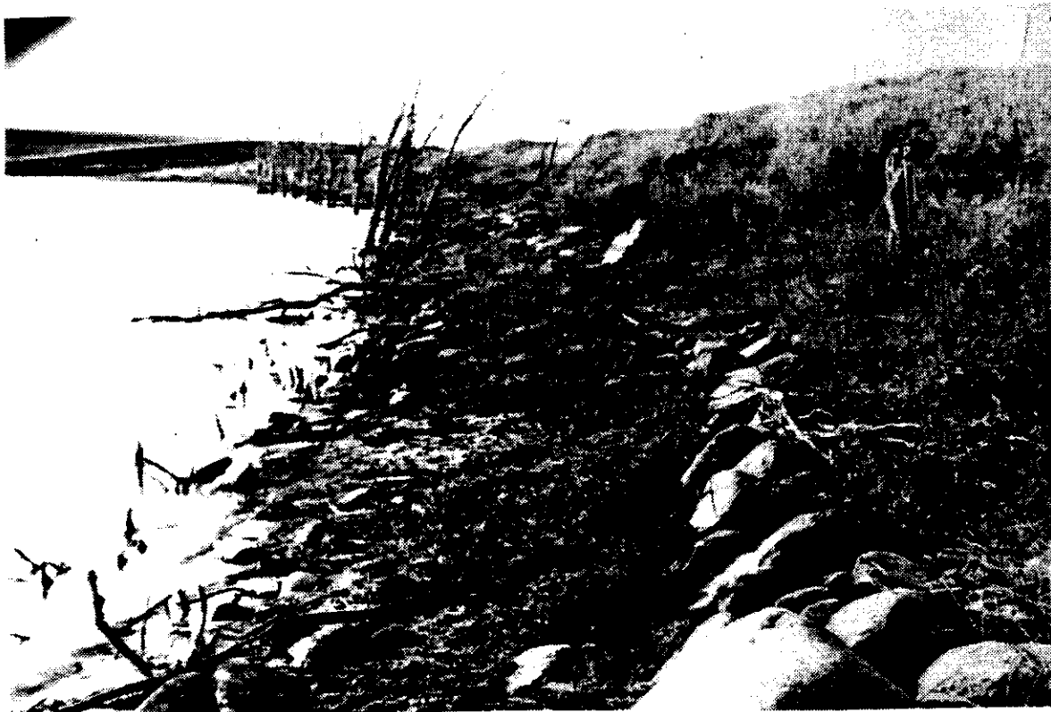
Photo # 5 Boulder line at elevation 1651.4 ft. msl.
