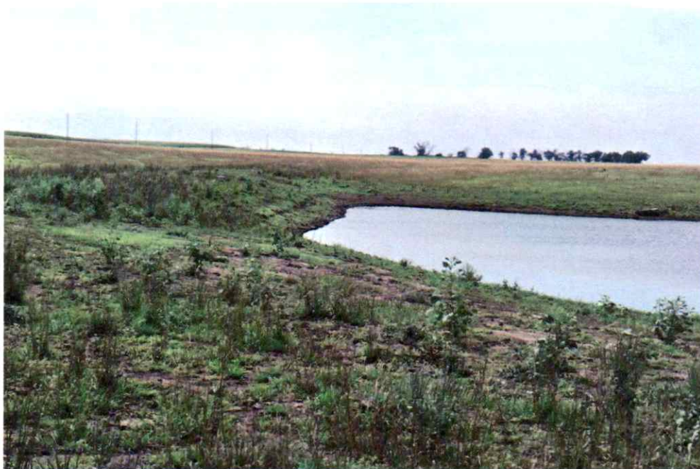
PIC 1. Looking south at upside of dam near the entrance to the secondary spillway.
