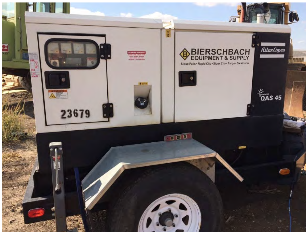
Photo 2: Well #1 aquifer test generator.
