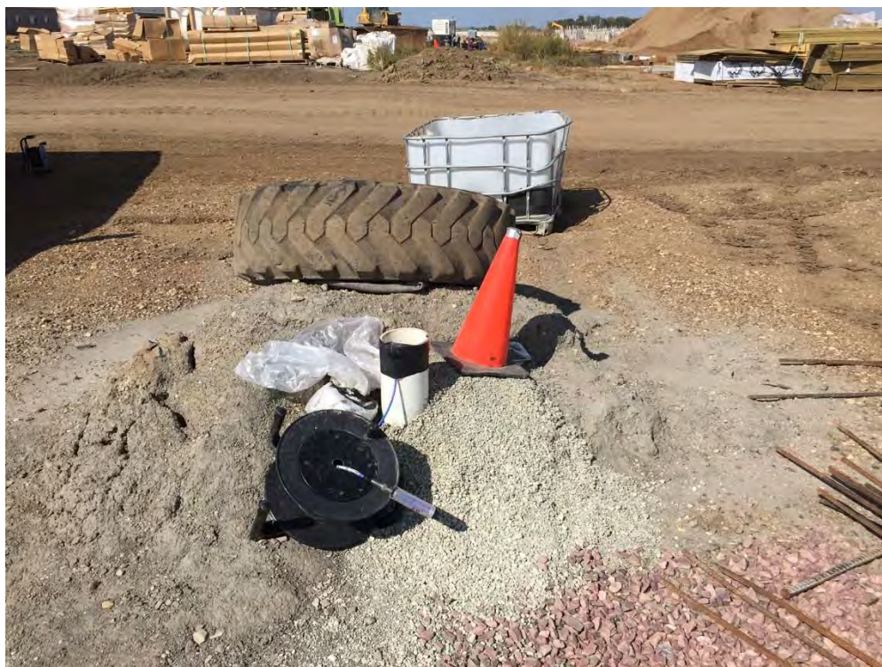
Photo 4: Well #3 looking north.
