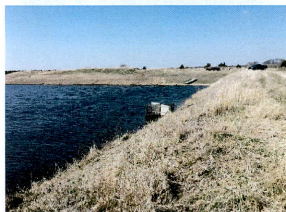
Looking N. Along the W. Side of the Dam
