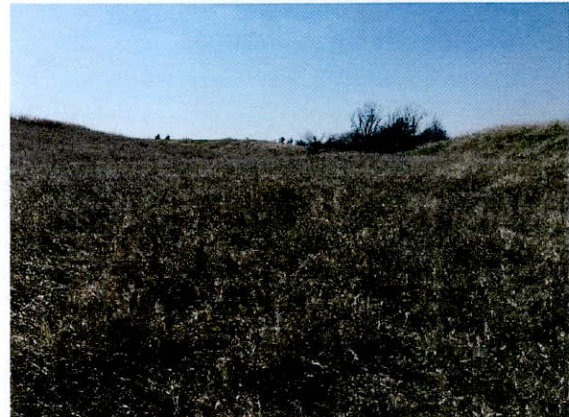
Looking West at the Overflow Spillway
