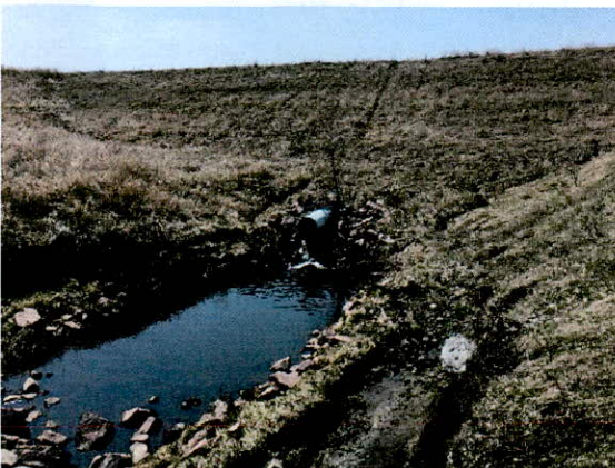
Looking West at the Discharge Pipe Outlet
