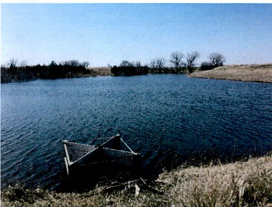
Looking West at the Outlet Structure
