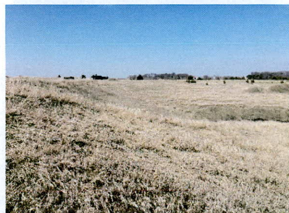
Looking NE Along the E. Side of the Dam
