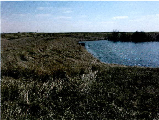
Looking S. Along the W. Side of the Dam
