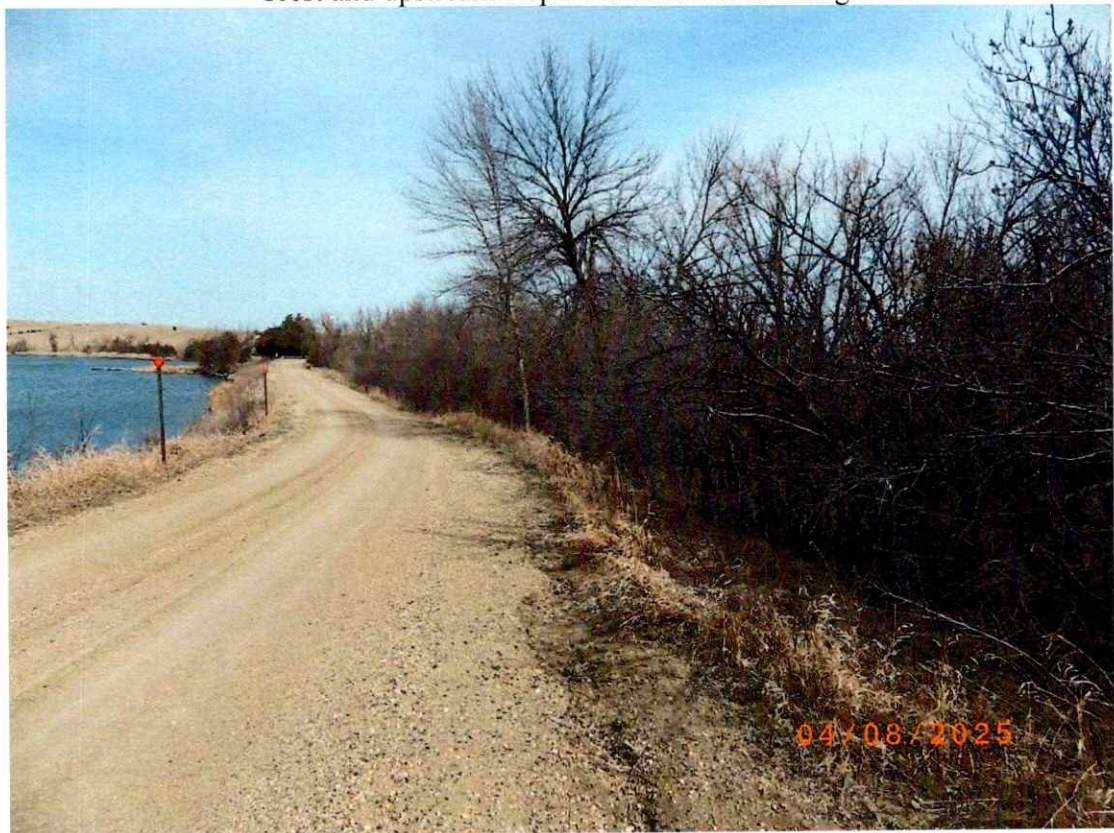
Crest and downstream slope. Note extensive tree cover on downstream slope.
