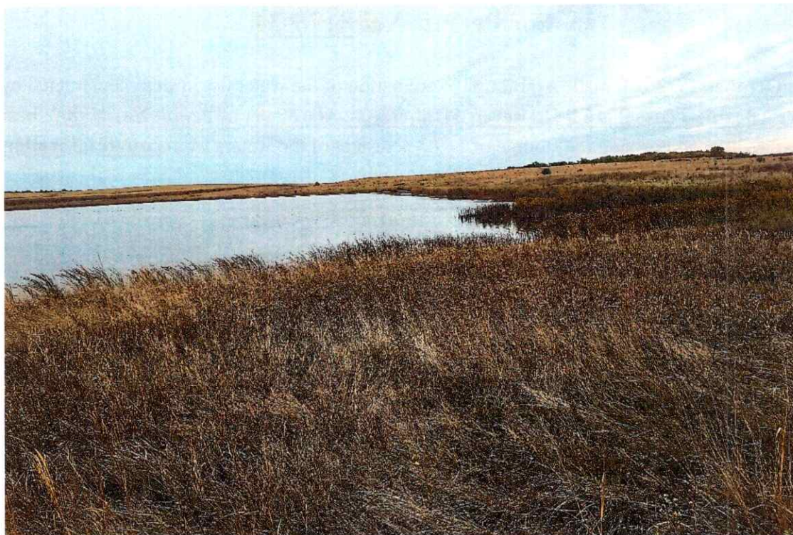
Looking southeast across the impoundment. The dam is to the right in the photo.
