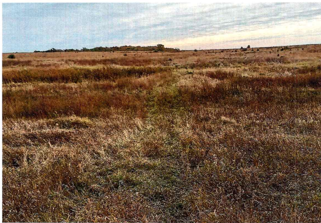
Looking south along the crest of the dam. Excellent vegetation makes it difficult to see the dam, but it is the light-colored mound in the center of the upper one-half of the photo. The emergency spillway is shown in the lower one half of the photo.
