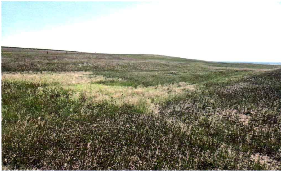
PIC 4. Looking south down the grassed primary (surface) outlet with excellent cover. Estimated to be about 35 feet wide at the outlet bottom.
