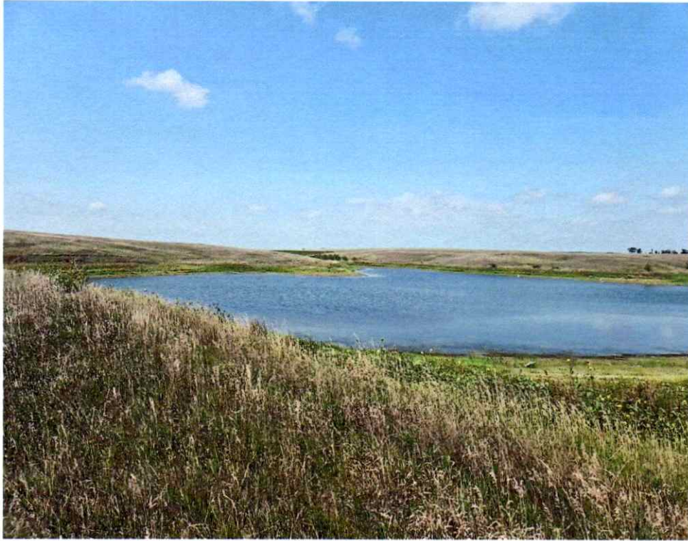
PIC #2. Looking west along the center line of the dam.
