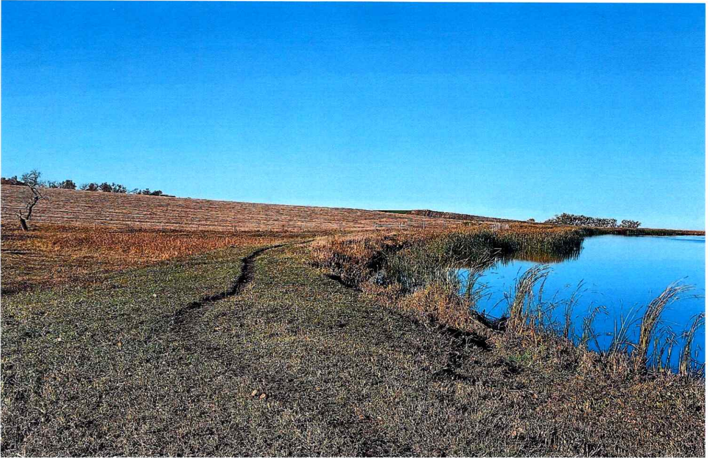
Looking SW across the small dam. Good vegetative cover but is grazed. No noticeable downside dam erosion. Some water-side dam erosion.
