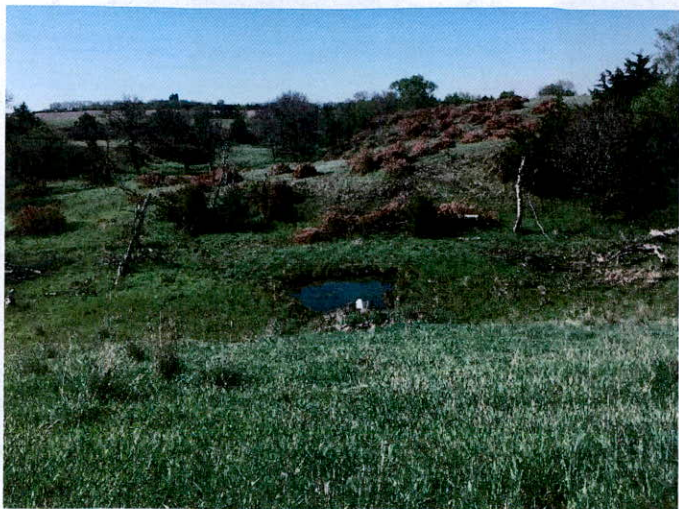
Looking South from the Center of the Dam at the Outlet Pipe Discharge
