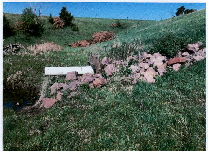
Looking West at the 12 Inch PVC Outlet Pipe
