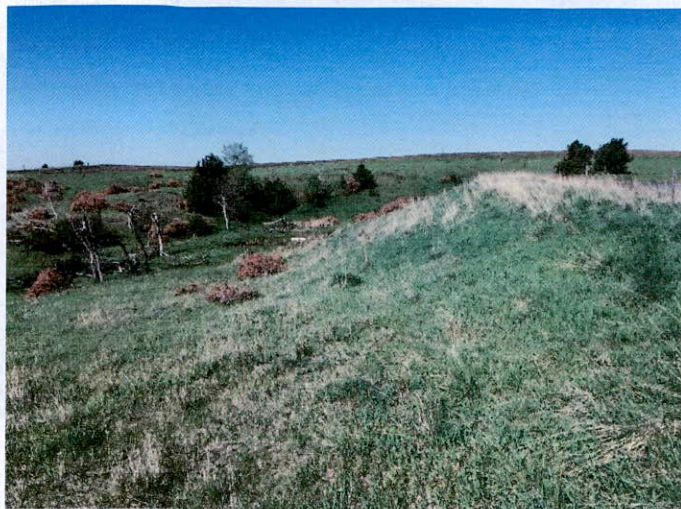
Looking West along the South Side of the Dam
