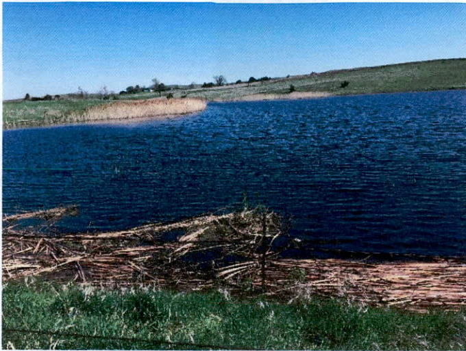
Looking North from the Center of the Dam at where the Pipe Outlet Should be Visible
