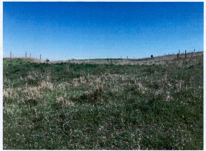
Looking North at the Auxiliary Spillway
