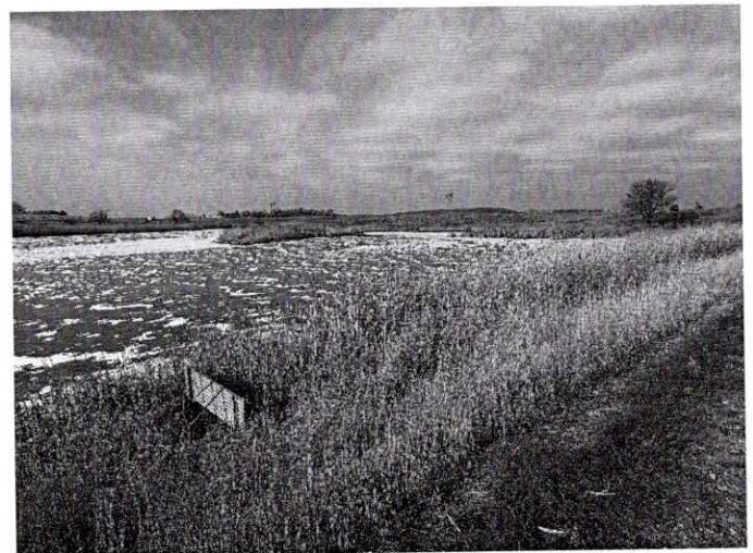
Looking west-northwest from the top of the dam at the lake and the 6' riser with a 36" CMP outlet pipe.
