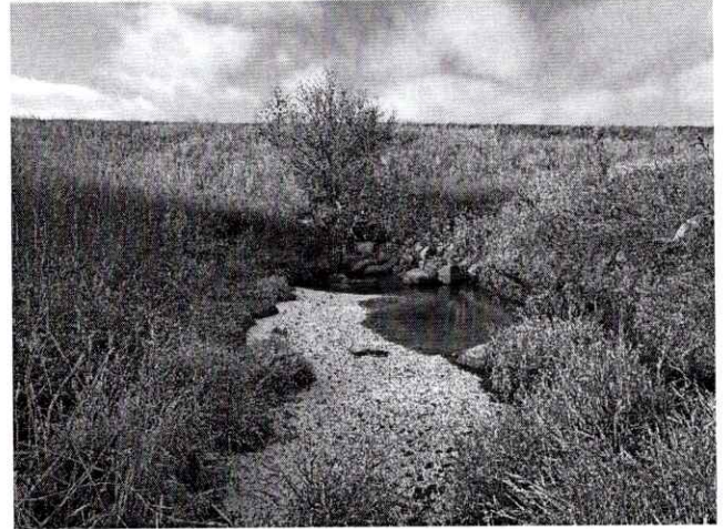
Looking west at the dam and discharge pipe outlet from the downstream drainageway.
