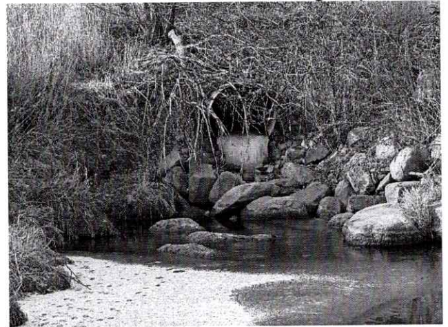
Looking west at the 36" CMP discharge pipe outlet.
