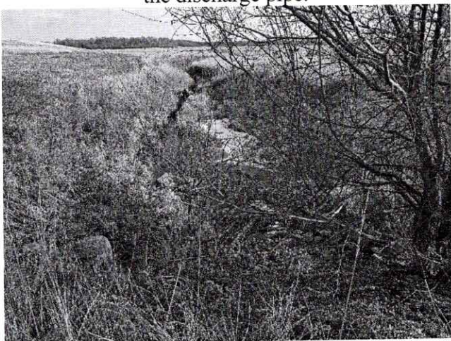
Looking east from just above the discharge pipe outlet.
