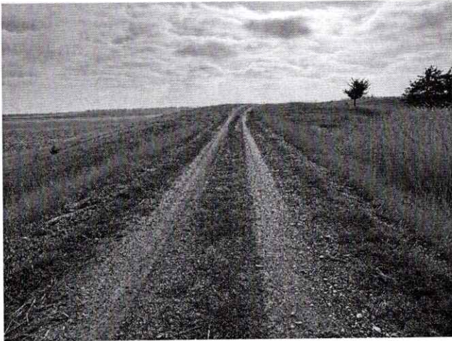
Looking south along the top of the dam from above the discharge pipe.
