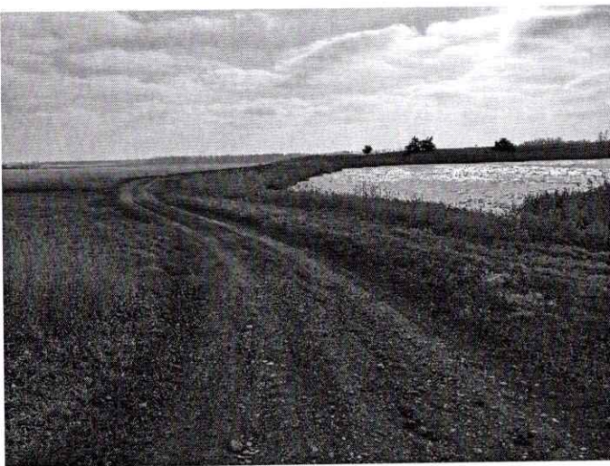
Looking south across the overflow spillway at the dam and lake.
