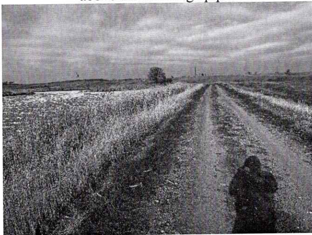
Looking north along the top of the dam from above the discharge pipe.
