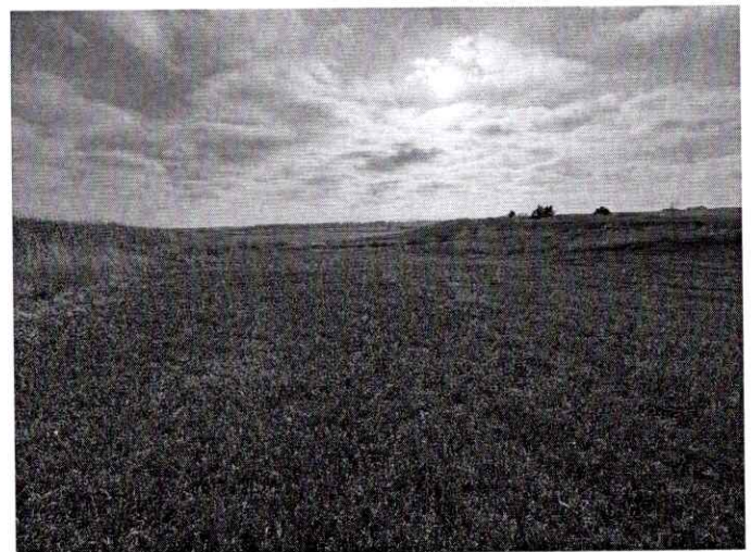
Looking south from the overflow spillway along the east side of the dam.
