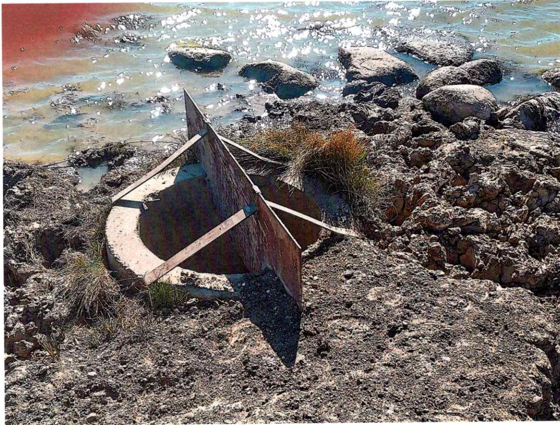
PHOTO #3. Shows the 30-inch concrete drop principal spillway with the anti-vortex plate. Also note the evidence of cattle hoof prints where they access the water for drinking purposes.
