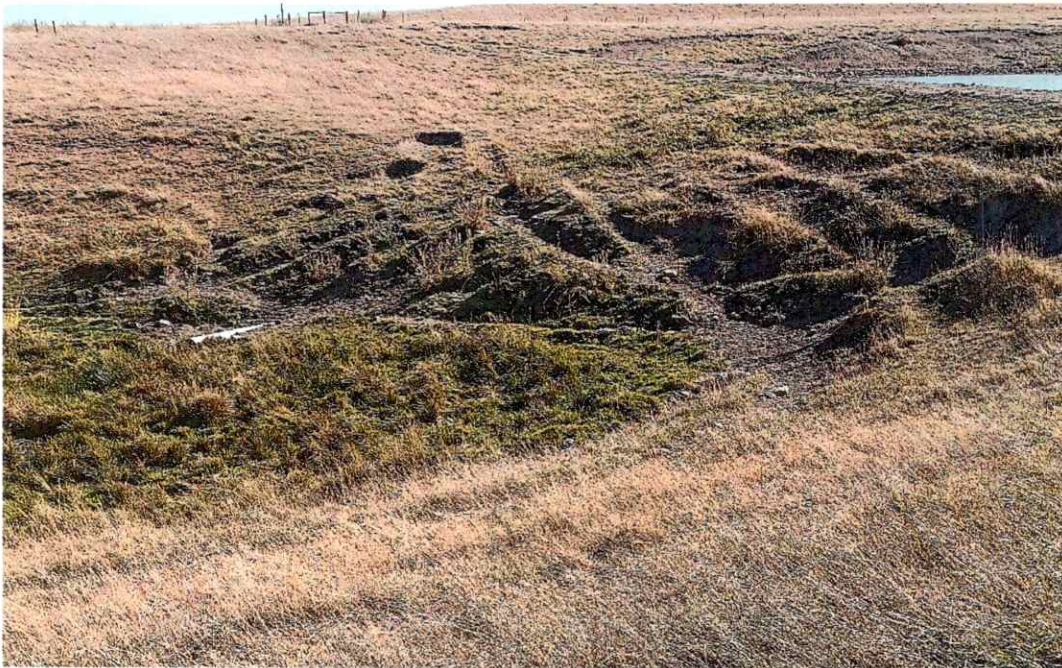
PHOTO #2. Looking southeast at the downstream side of the dam showing some loss of vegetation where cattle travel, but in general there is good grass on the downslope. Did not see any serious erosion problems beyond a limited area shown in the photo. The white pipe is the principal spillway outlet.
