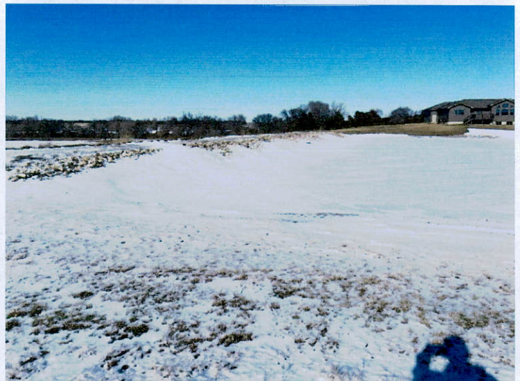
Looking North-Northwest at the Dam and Riprap
