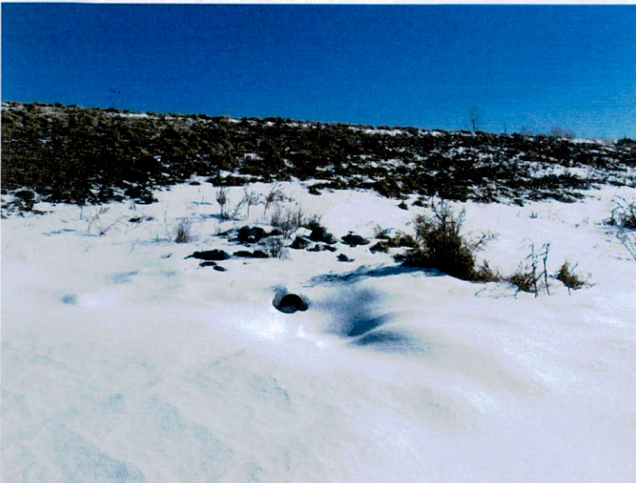
Looking East at the Outlet Pipe
