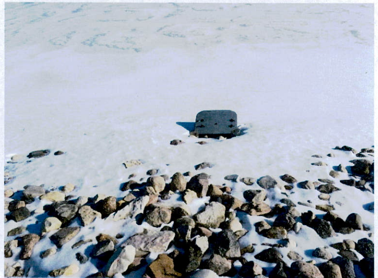
Looking East at the Overflow Pipe
