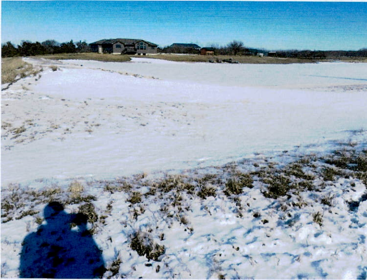
Looking Northeast at the Dam and Spillway
