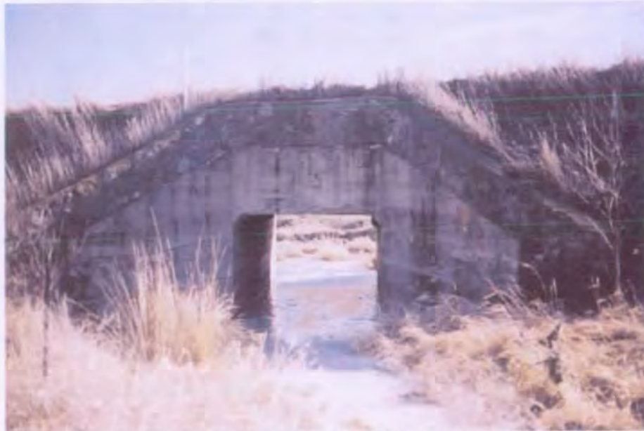
Photo 1 Box Culvert under 271 st Street (April 2005)
