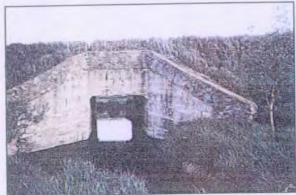
Pool under bridge
