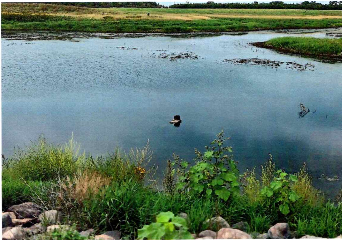
PIC 2. Looking west at the inlet from top of the dam. Note the riprap on the upper face of the dam.
