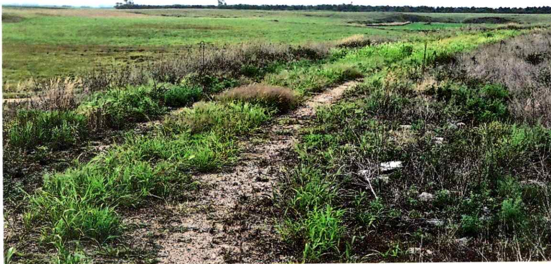
PIC 6. Looking downstream from the dam.
