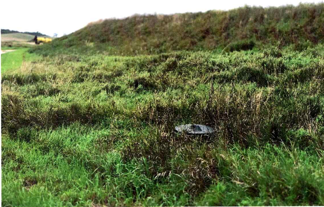
PIC 5. Looking at downslope of the dam. Note excellent grass cover and steep downslope.
