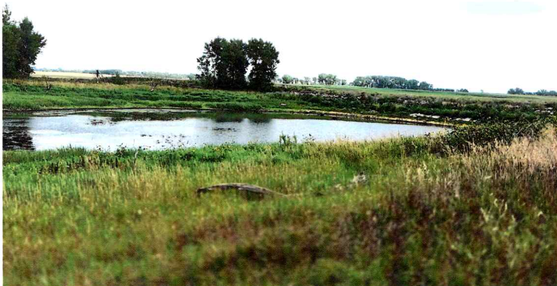
PIC 3. Looking northeast towards the dam from the east edge of the secondary spillway.
