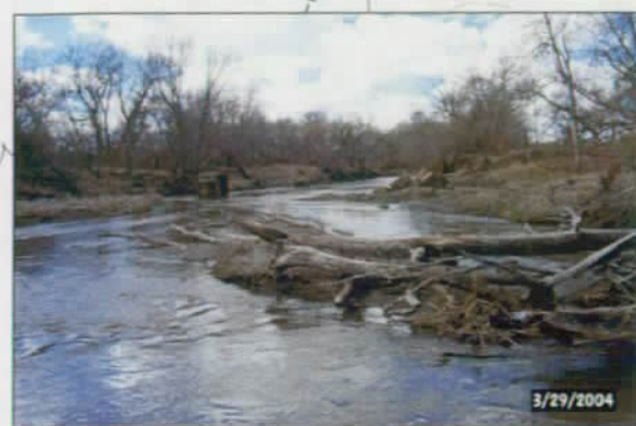
PHOTO 2 VIEW LOOKING DOWNSTREAM
