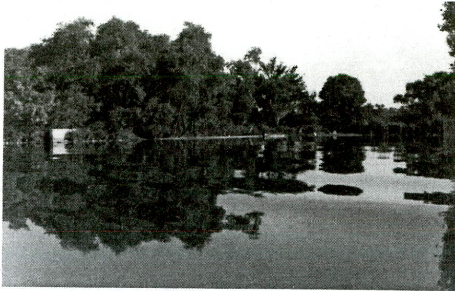
PHOTO NO. 11 Outlet Structure 134 feet wide Elevation----1575.2 ft. msl
