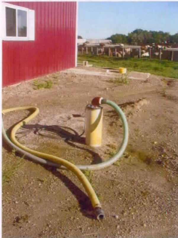
Picture of well taken September 10, 2007
