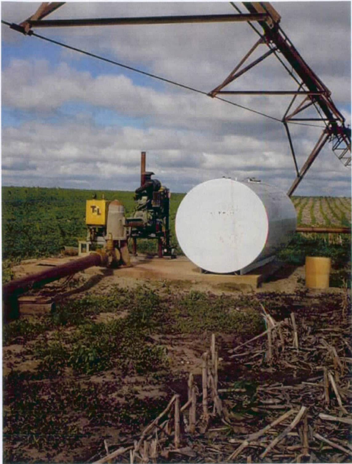
Well, motor, center pivot and fuel tank at pivot point for Water Permit No. 6332-3
