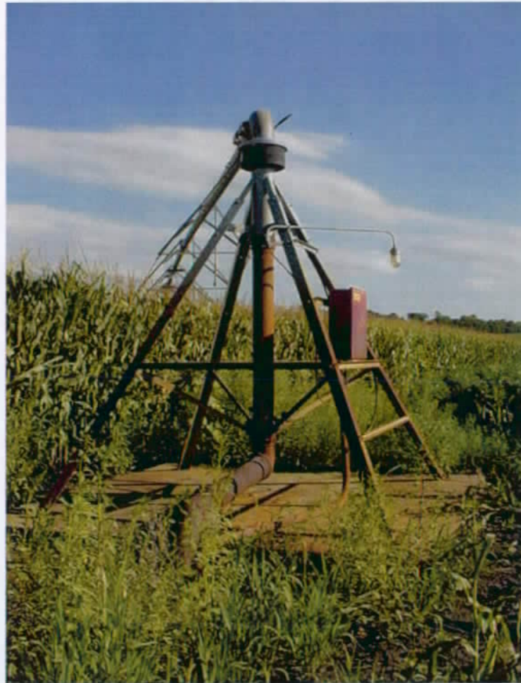
Pivot Point for System authorized by Water Permit No. 6302-3 (this water permit should be incorporated with Water Right No. 3197-3)
