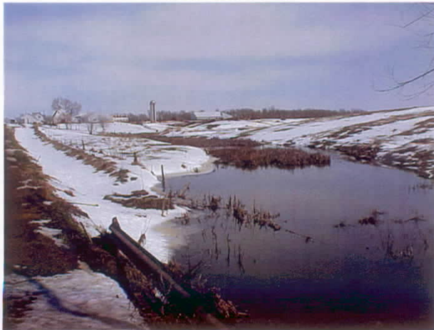
398 th Ave. 15 foot Bridge & Upstream Channel
