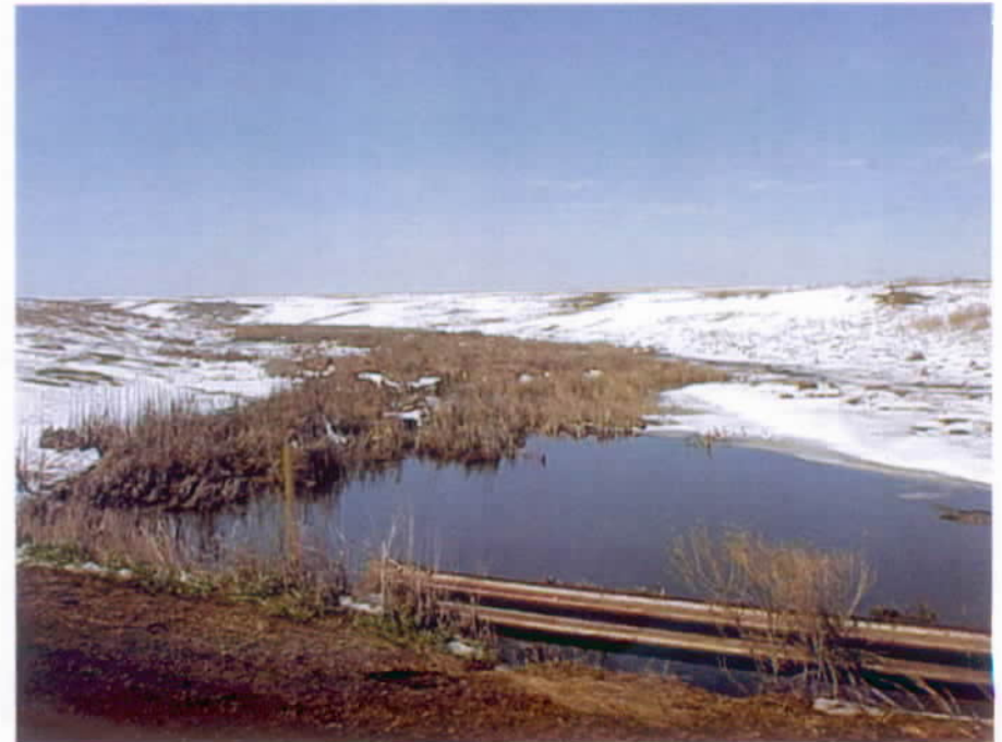
398 th Ave. 15 foot Bridge & Downstream Channel
