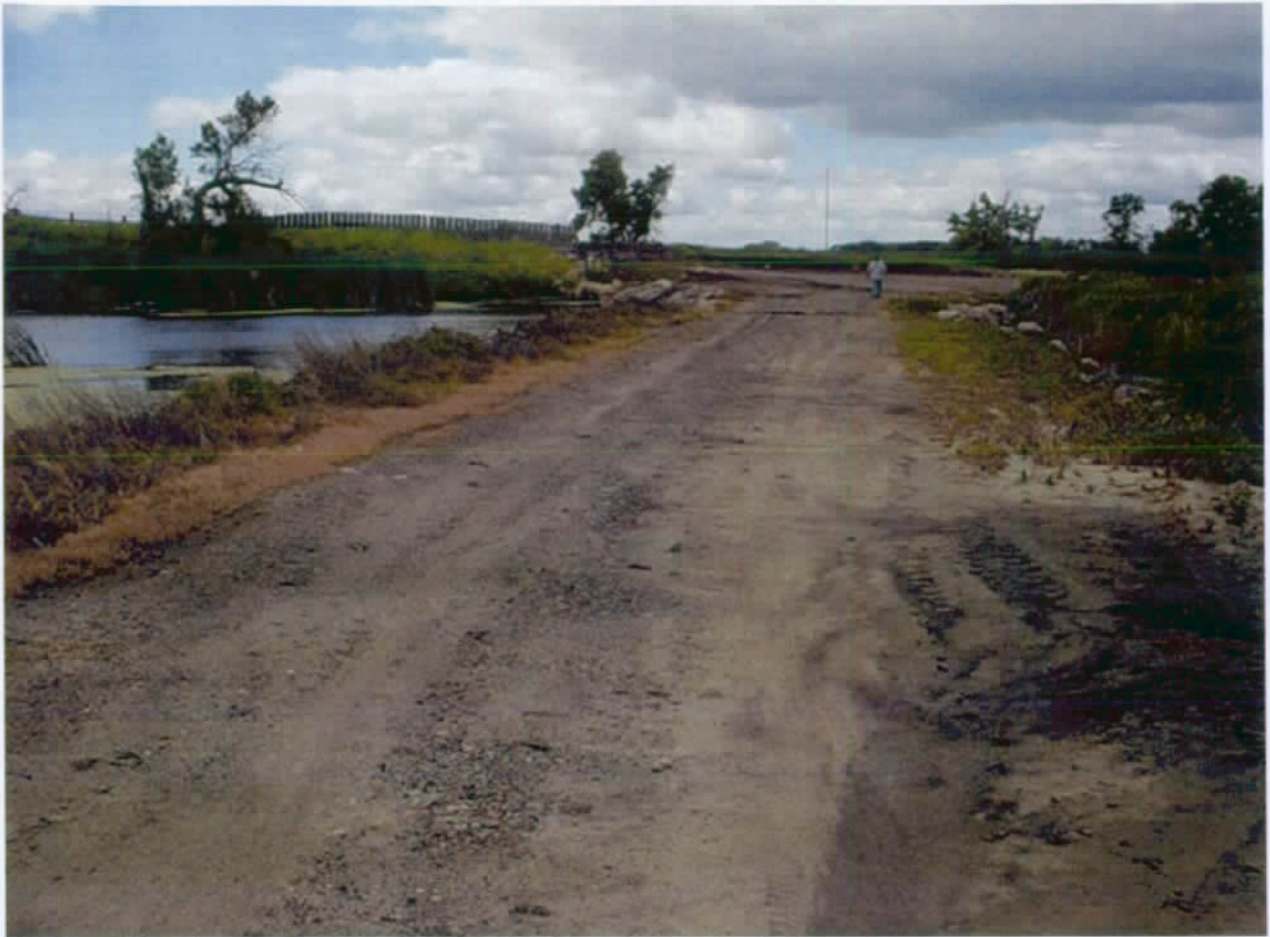
Picture of the dam taken from the north looking in a southerly direction.
