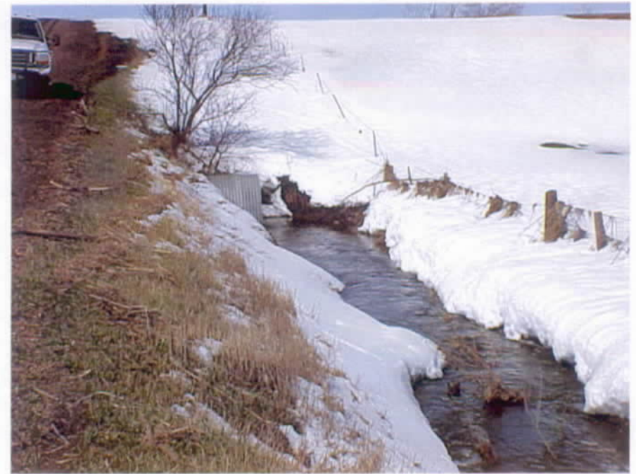
185 th St. 4 foot CMP Culvert
