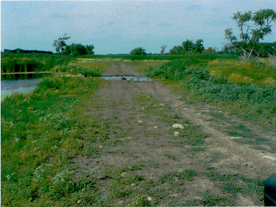
Figure 2 – Small dam located in SW¼ of Sec 10 T114N-R62W
