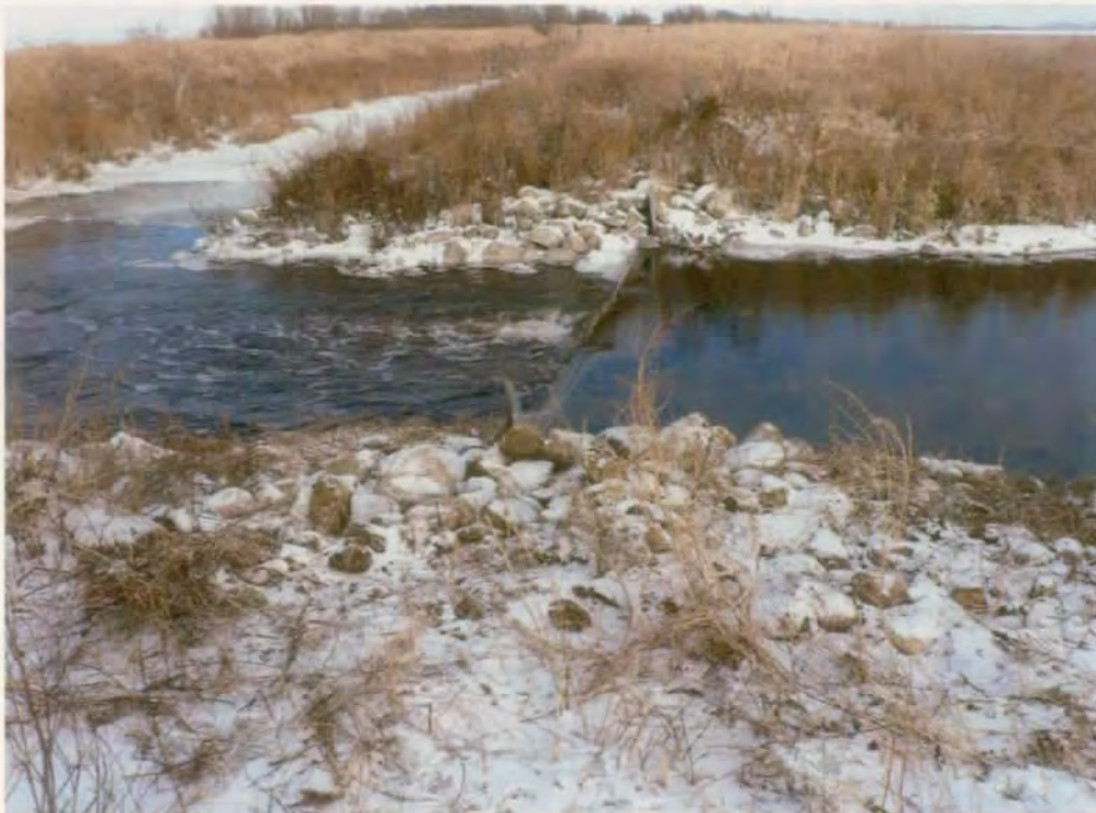
December 2008 – Repaired breach at Putney outlet structure SW ¼ Sec 18 T124N-R62W
