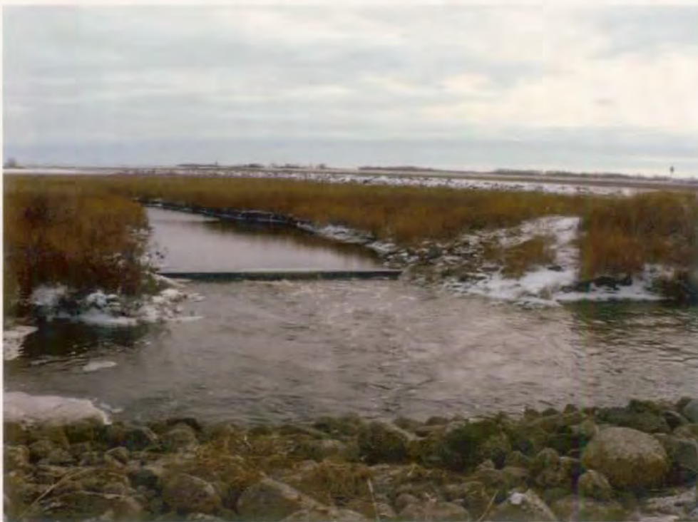
December 2008 – Repaired breach at Putney outlet structure SW \frac{1}{4} Sec 18 T124N-R62W
