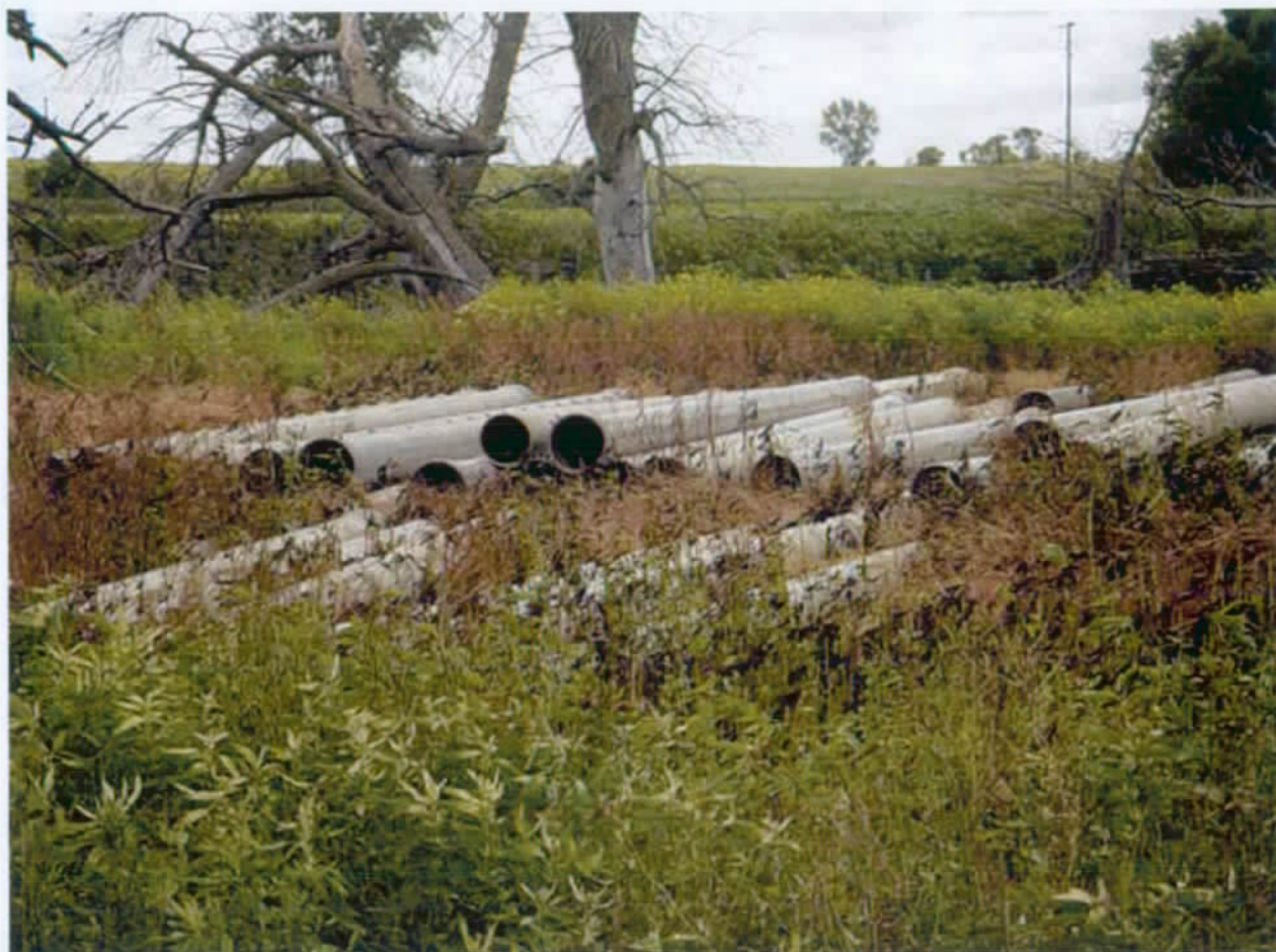
Aluminum pipe on site at pump station No. 3
