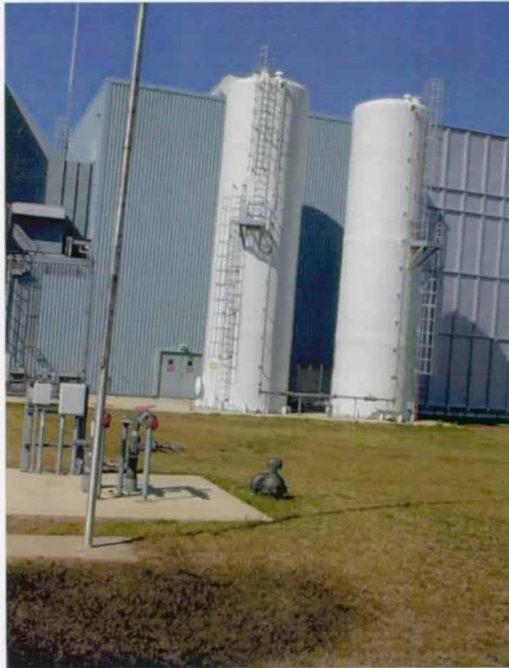
Primary well with storage in background
