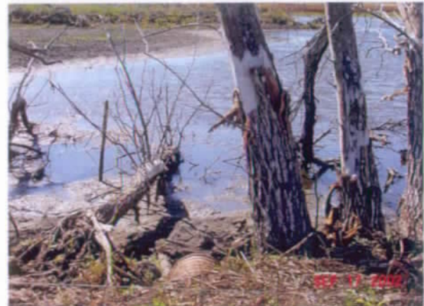
Water level below culvert outlet thru road
