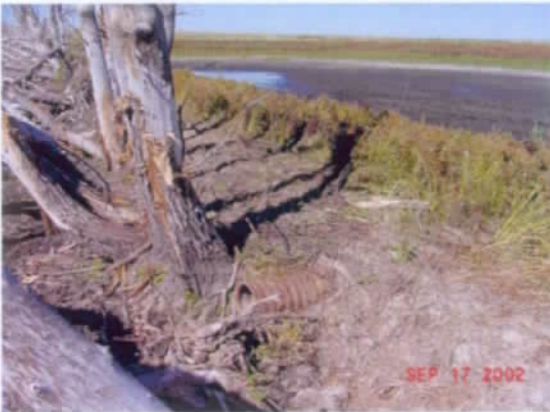
Culvert outlet through section line road
