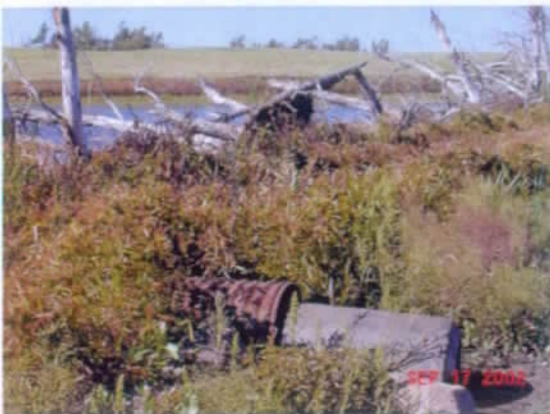
Culvert inlet through section line road
