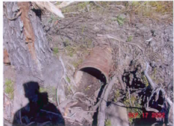
Closeup of outlet through section line road
