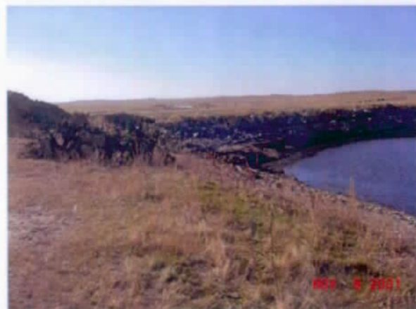
Dam embankment – dirt work to lower water
