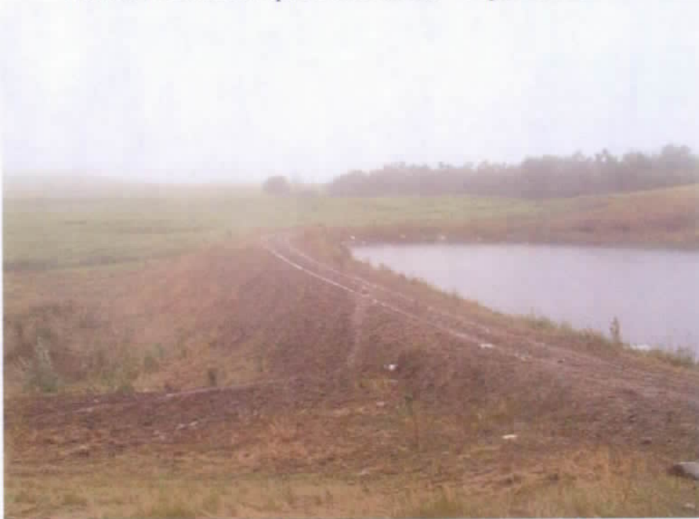
Picture showing the downstream side of the dam embankment looking towards the west. Outlet of the 24 inch culvert is in the lower center of the picture.
