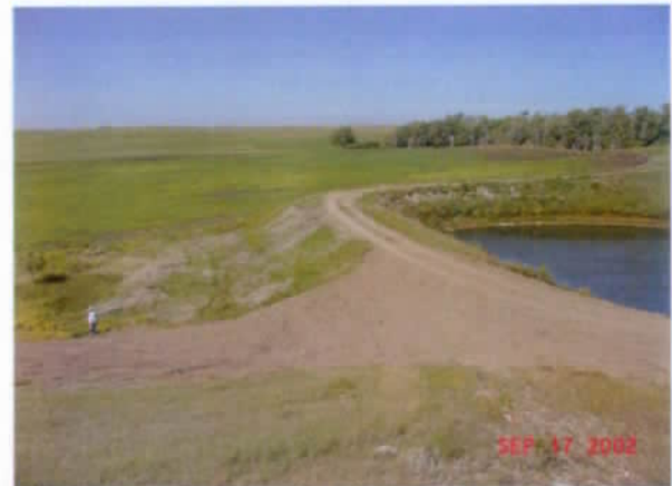
Dam embankment - dirt work to lower water
