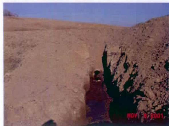
Downstream exit from 18 in culvert
