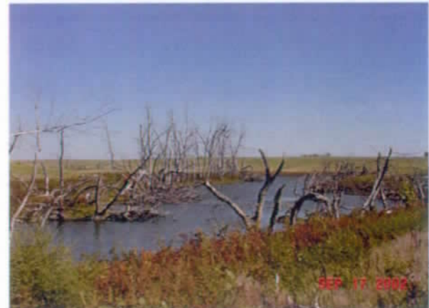
Upstream closeup of dam pool
