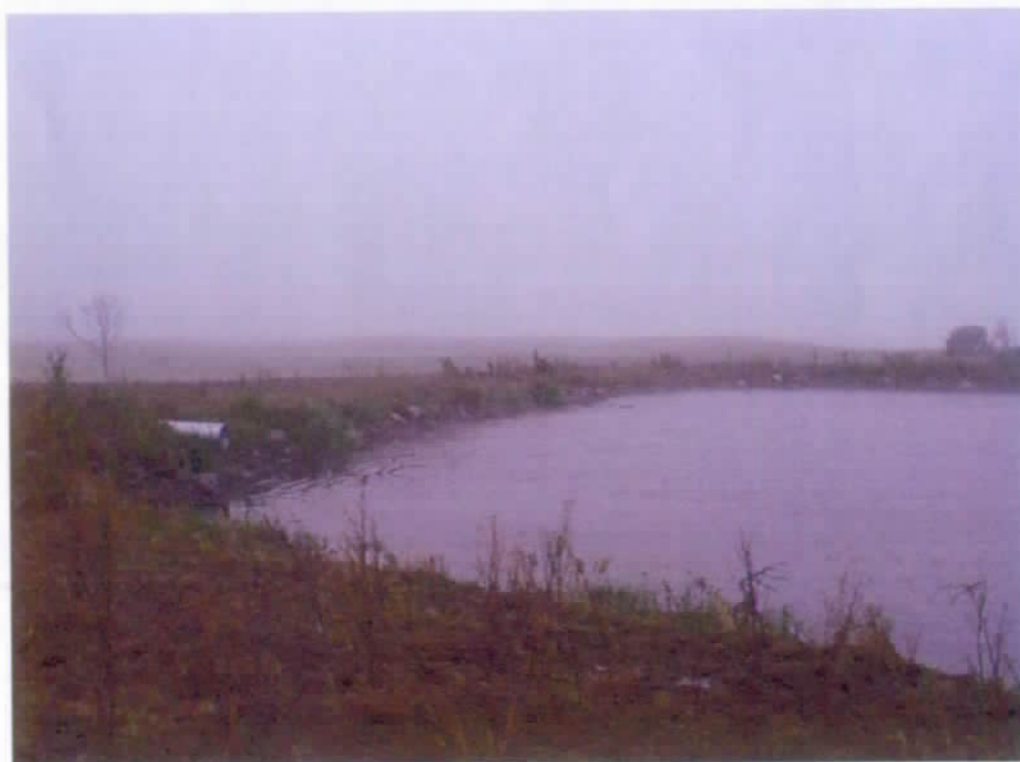
Picture of the upstream side of the dam embankment looking towards the west.
