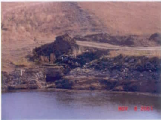
Entrance to 18 inch culvert spillway
