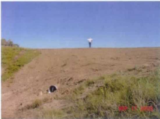
Outlet of the 24 inch culvert spillway
