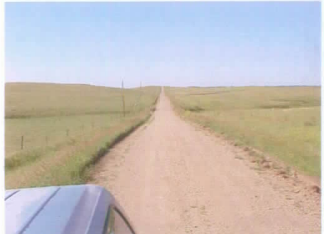
A12: Looking south to where the drainage crosses road between sections 25 and 26-116N-71W - approximately 1.5 miles below the dam
