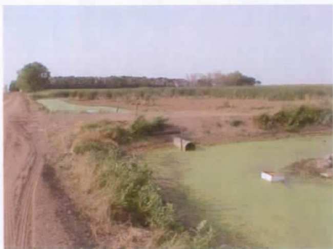
B1: Looking south (downstream) from near corners of sections 35, 36-116N-71W and sections 1, 2-115N-71W -- culvert now exposed due to lower water levels
