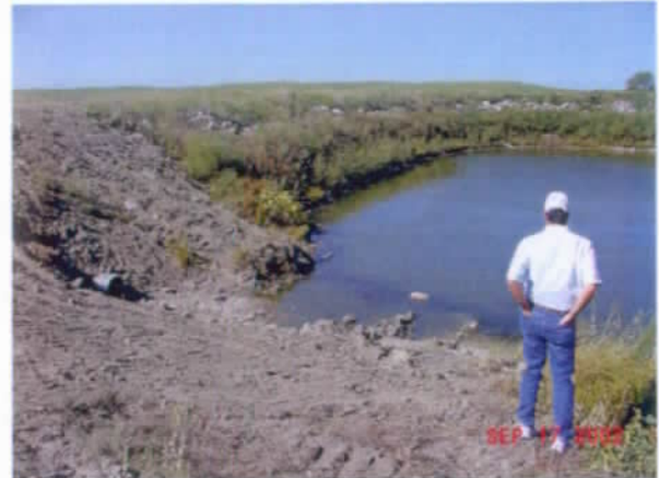
Upstream embankment with inlet on left
