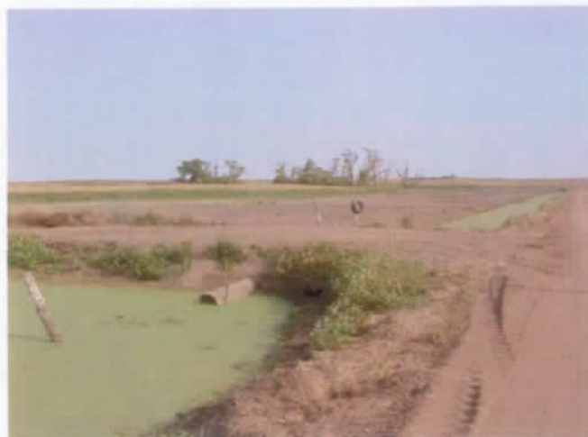
B2: Looking upstream near corners of sections 35, 36-116N-71W and sections 1, 2-115N-71W -- opposite end of culvert shown in photo B1
