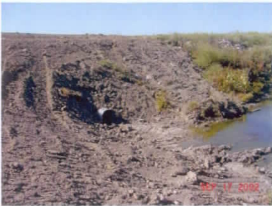
Inlet to 24 inch culvert spillway
