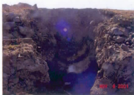
Upstream entrance to 18 in culvert
