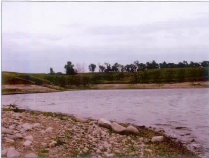
Intake Bay (North - Toward Spring Creek Road)
