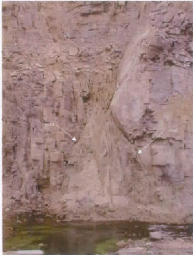
Figure 1. Zone of Uncemented quartzite where inflow was encountered
