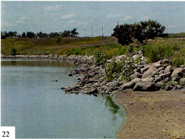
7-26-00 - Dark water mark on rip rap elev. 1248.6 fmsl. W½ SE¼ and E½ SW¼ Sec. 23-T113N-R61W
