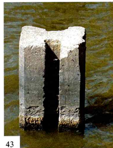
7-20-00 - Water mark on old concrete bridge pile elev. 1248.2 fmsl. SE¼ NE¼ Sec. 25-T113N-R61W
