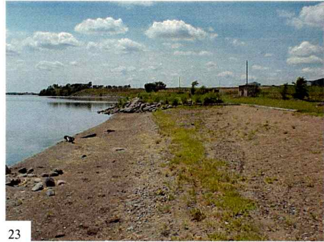
7-26-00 - Beach cross section, top of washed pebbles elev. 1249.6 and top of swimming beach elev. 1251.4 fmsl. W½ SE¼ and E½ SW¼ Sec. 23-T113N-R61W
