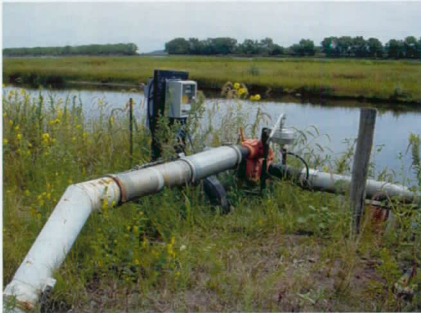
Missouri River diversion point located in the NW \frac{1}{4} SE \frac{1}{4} Section 1, T91N, R52W
