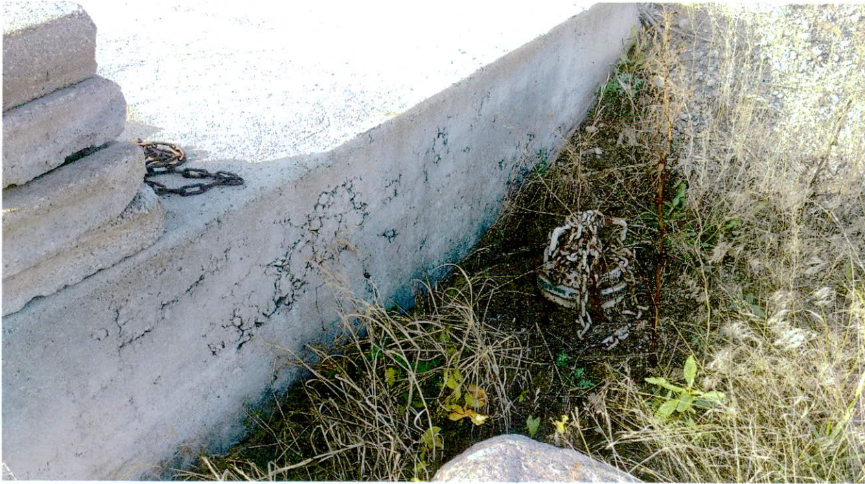
Picture 2. Inlet to pipeline running to section 26.
