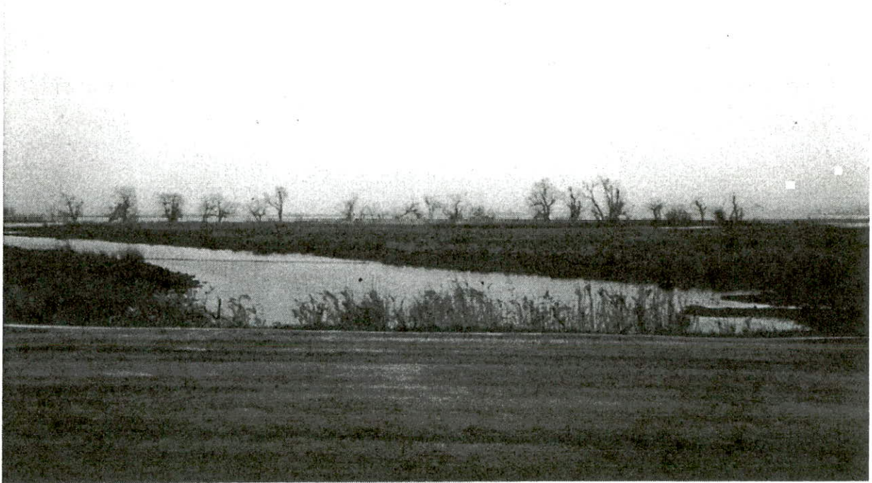
Photo No. 1: Round Lake outlet channel upstream side of the culverts.
