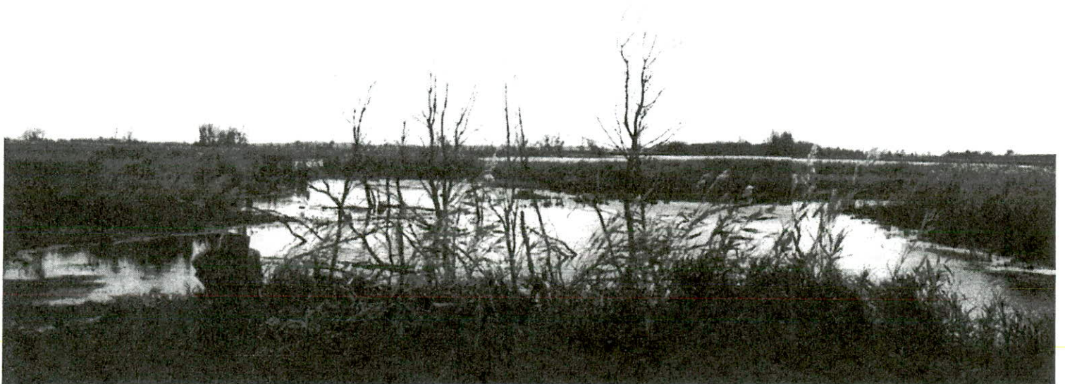
Photo No. 4: Upstream side of the culvert from Bullhead Lake to Round Lake. Slough between Bullhead and Round lakes.
