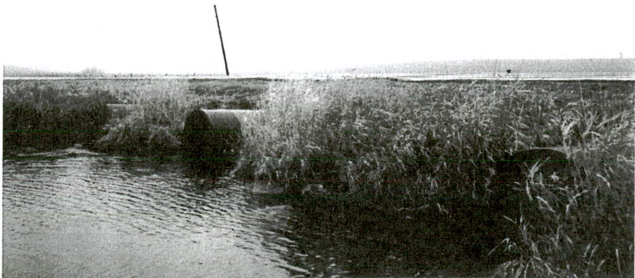
Photo No. 2: Five foot diameter Culverts in Round Lake outlet channel; overflow elevations of 1857.11, 1857.47, and 1857.83 fmsl.
