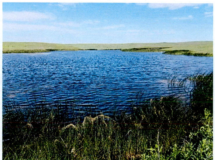
pool and front face of dam in foreground
