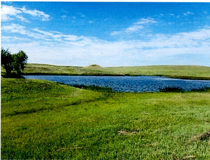
reservoir pool, spillway in foreground, embankment on left
