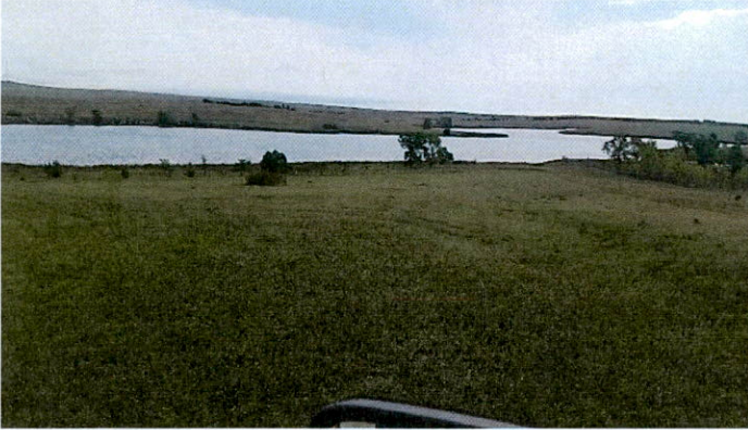
Reservoir viewed from northwest
