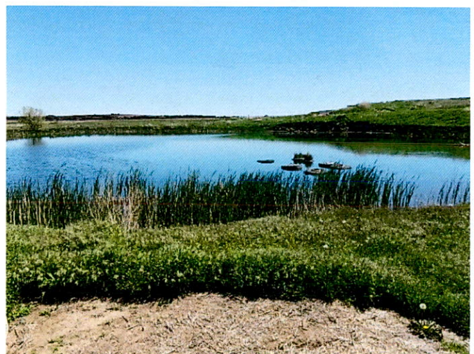
Clean water storage reservoir
