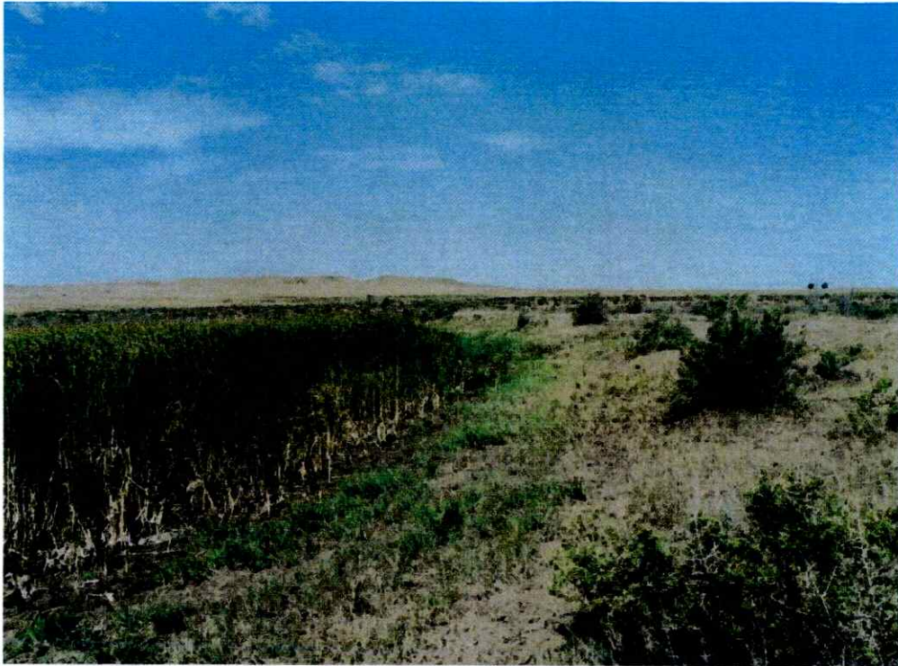
Figure 2 - Photo Location A- Diversion dam on Coal Creek located in the NE \frac{1}{4} NE \frac{1}{4} of Sec 26 T10S-R2E.
