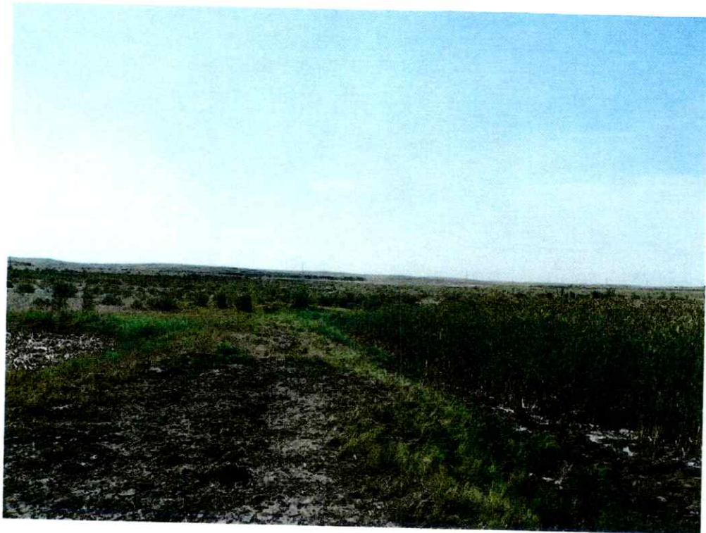
Figure 4 - Photo Location B- Diversion dam on Coal Creek on the right and top of the main ditch/dike on the left for Water Right No. 28-2 (Nos 28A-2 and 28B-2) Creek located in the NE \frac{1}{4} of Sec 26 T10S-R2E.
