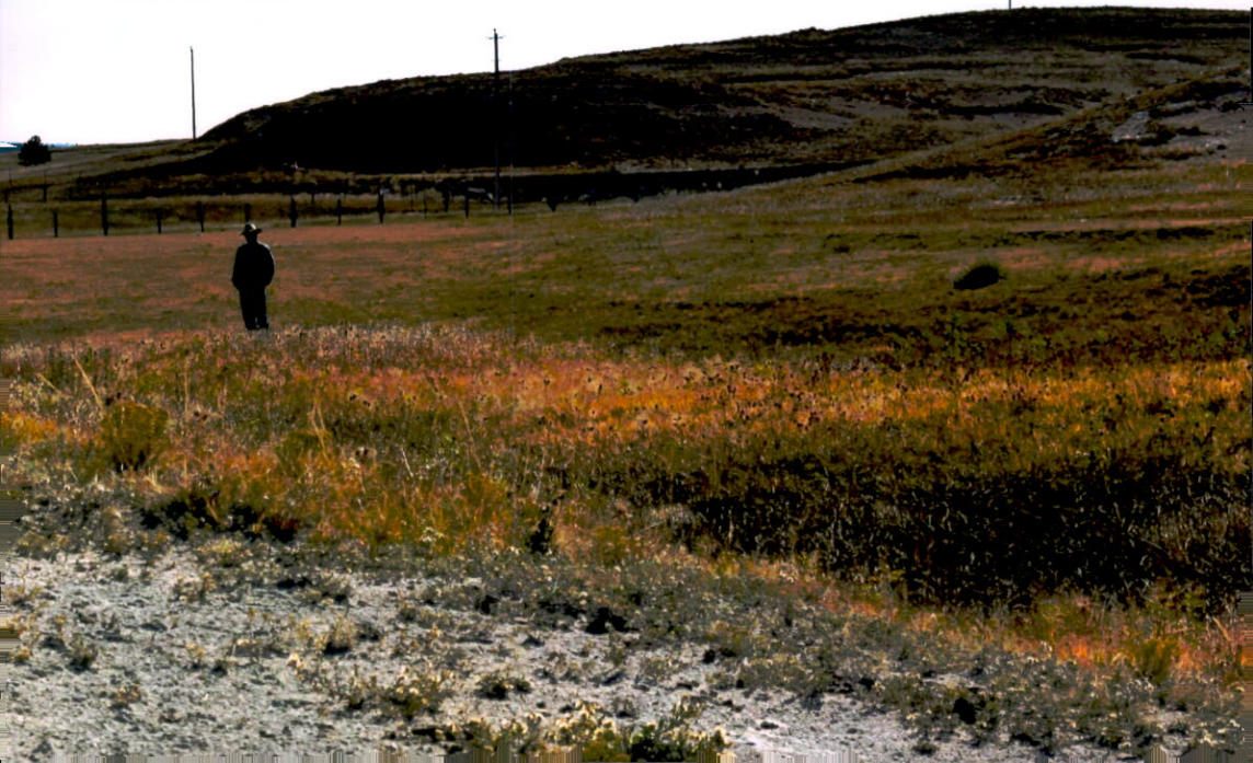
Dan Stearns standing near the spillway - West Fork Coon Creek Dam - 10/09/2022
