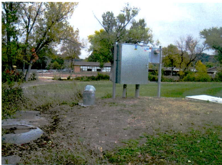
Photo 1--Image of Arrowhead's subterranean pump house adjacent to Rapid Creek with Meadowbrook School in the background.
