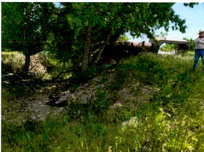
Spillway channel allowing partial return of diverted flow back to creek. Concrete box culvert section at upper right to be used to rebuilt control section.
