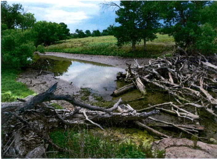
View from crest of Diversion Structure looking upstream on Spring Creek
