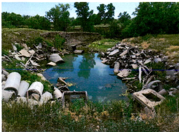
Spring Creek diversion outlet
