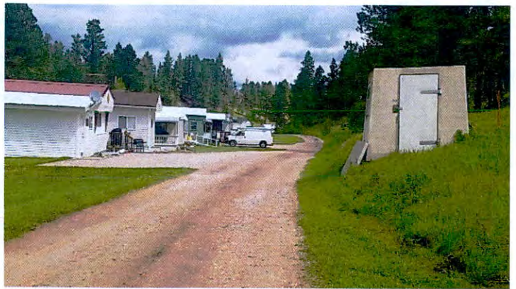
Well #2 pump house
