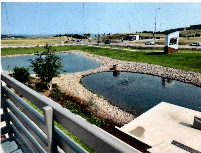
Storage pond with aerator
