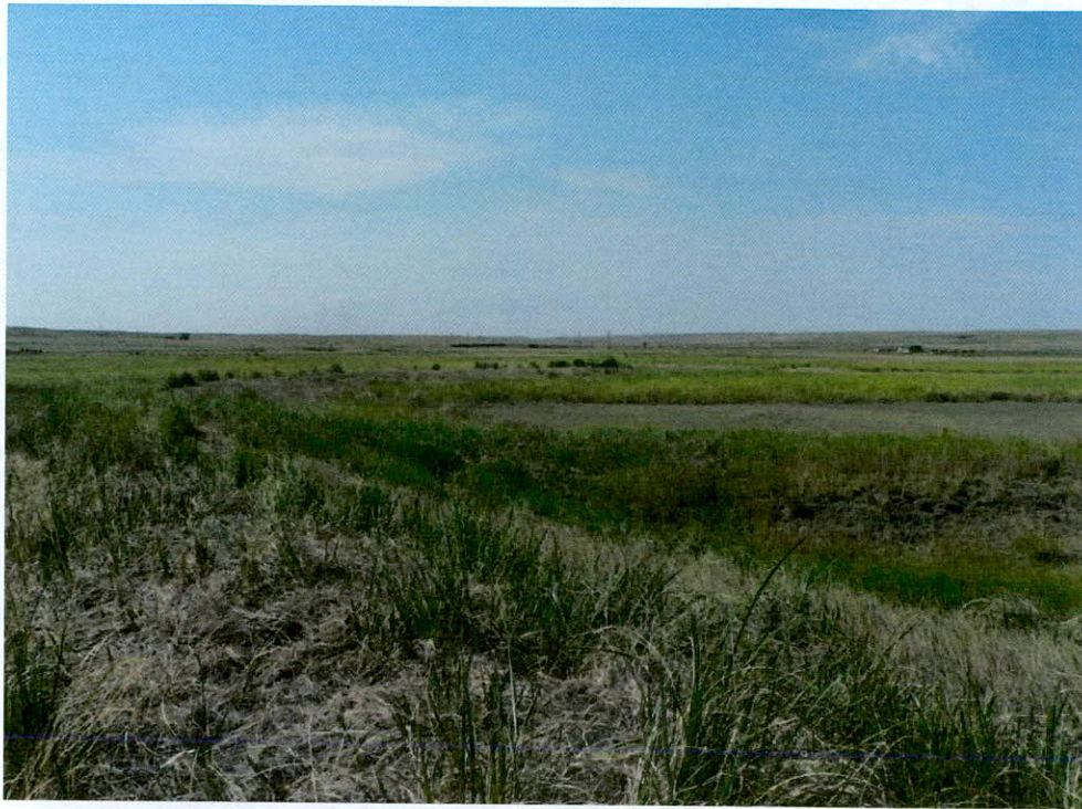
Figure 6 - Photo Location D - A spreader dike to intercept runoff and disperse the water for irrigation located in the NW \frac{1}{4} SE \frac{1}{4} of Sec 24 T10S-R2E.
