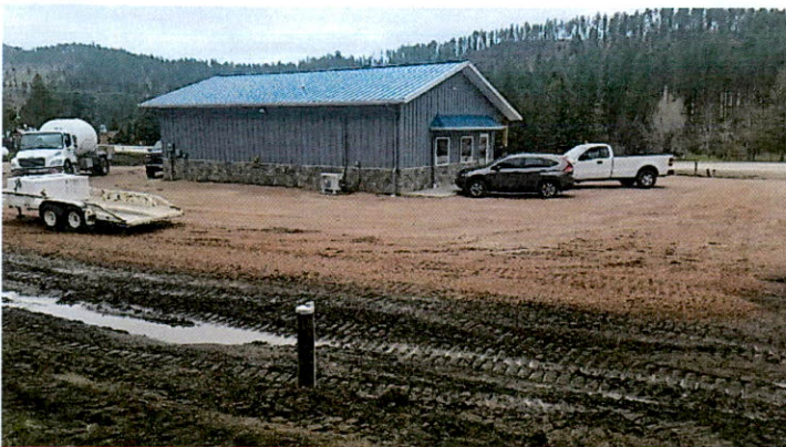
Well and Nelson Oil Building
