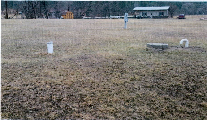
Forty Oaks Ranch Subdivision well and pit with one of the homes in background
